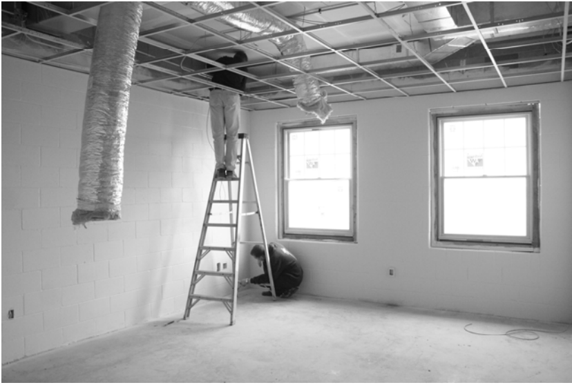
Work on communications system
